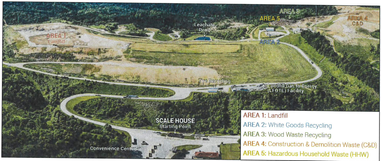
Figure 1-1: Buncombe County Solid Waste Management Facility
